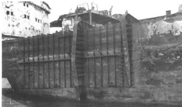
Fig.8. The path (7×14 m) welded with semi-automatic welding
