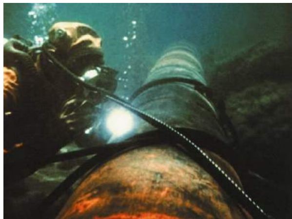
Fig.6. Wet semi-automatic welding of pipeline
