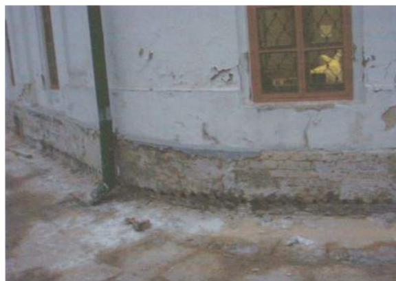
Fig.21. Drilling holes in the basement facade
