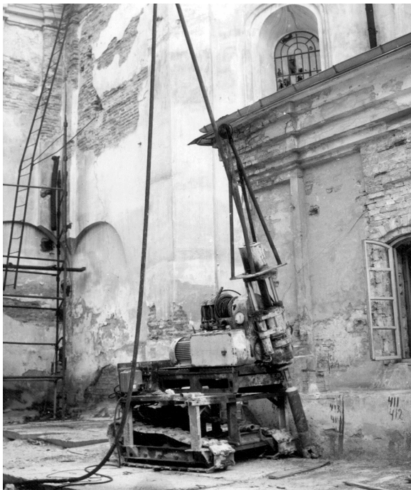
Fig.12. Drilling machine СКБ-4Е
