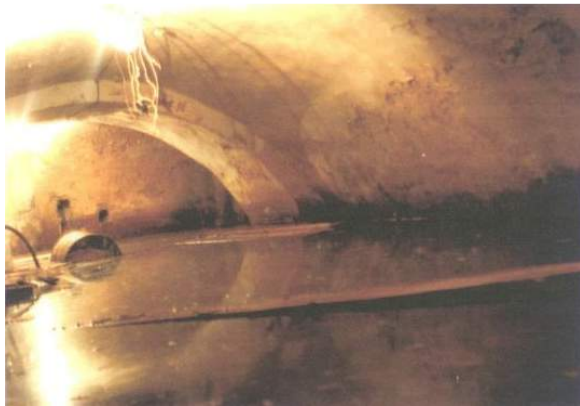
Fig. 16. Basement before the work
