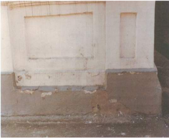
Fig.17. Basement before the work
