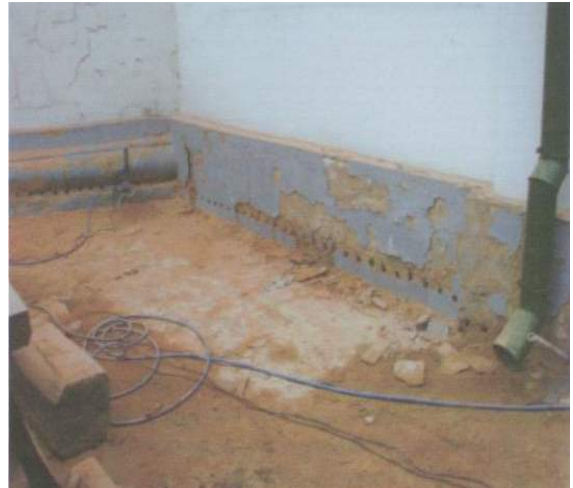
Fig.18. Drilling holes in the basement facade
